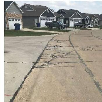
This is the oldest section of Stonewater streets and the most damaged. After nearly 20 years of wear from construction equipment, trucks and cars, it's time to have it replaced.
