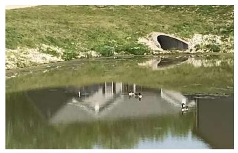
When work began on Phase 2, contractors converted a low-lying area along Rolling Stone into a retention pond. The basin holds runoff from Living Stone, Watering Stone and Rolling Stone, as well as from both sides of Festus-Horine Road.
