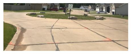
Stonewater Drive replacement will be beyond the roundabout and will involve five slabs. This section is original to the subdivision and in use for more than a decade. Vehicular traffic and access by construction equipment took a toll.
