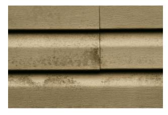
Remember, the accumulation of dirt and dust is one of many reasons why mildew grows on your vinyl siding. Others, according to GoldEagle.com, are excessive moisture (not just rain; consistent wet spots from poor drainage, dripping faucets or air conditioner condensation), and lack of sunlight (hence, the north side of homes or areas in lengthy daily shade).
